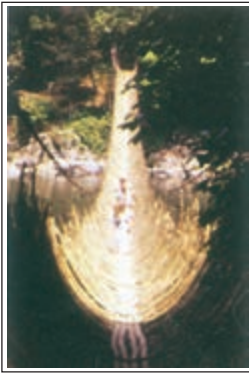
Figure 6.7 : Rope Bridge (Arunachal Pradesh)
